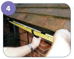
Mark the position of the fascia brackets, spacing them no more than 1000mm apart (400mm in areas of heavy snowfall) and no more than 150mm from any angle or stopend.
