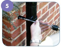
✓ Fit the pipe clips to the downpipe and screw them into the wall.
