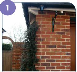
Using a plumb line, mark a vertical line on the wall from the outlet to the drain.
