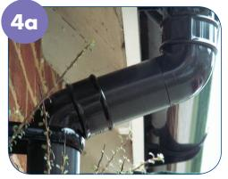
Working from the top downwards, install the downpipe. If additional lengths of downpipe are required, join using a socket and pipe clip.
