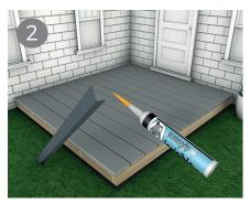
Once the corner trim is cut to size, you can use sumogrip adhesive along one or both sides of the corner trim and attach to the edge of the decking. To allow for expansion you may wish to only glue the top edge to allow for some movement.
