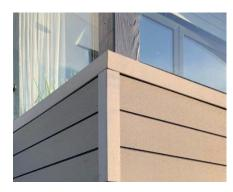
To use wall cladding as a fascia, you will need to ensure you have suitable joists behind to secure the wall cladding onto, then simply screw through the lip of the wall cladding board and install the next board on top. This can be done in a vertical or horizontal pattern (see wall cladding installation guide for more information).
