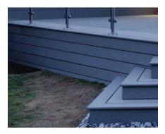
To use decking boards as a fascia, you will need to to ensure you have suitable joists behind to secure the decking boards. Measure and cut the board to the desired size, you can then install these using the t clip system in a vertical or horizontal pattern.
