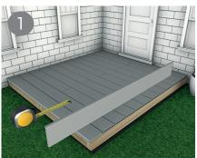
Measure the edge of the decking area to obtain the length required, skirting trim can be cut to size as needed. If you need a longer length than 2.2m simply butt the two skirting edges up together.
