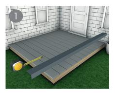
Take the corner trim and measure the length of the area its going to be fitted on to. Corner trims can be cut and worked just like timber so can be cut to desired size. If placing two trims side by side, simply butt up together.
