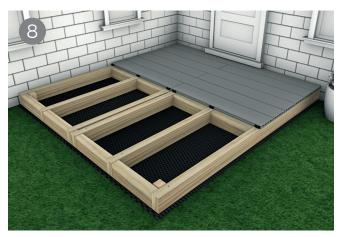
Fit your next board by sliding it onto the T-Clips used to secure the first board and fitting another set of T-Clips to secure the opposite side of the board, again one T-Clip for each supporting joist. Follow a similar process to fix subsequent boards.
