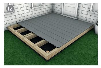
Having fastened your boards all that remains is to tidy up the sides of your new deck with our composite skirting or fascia boards which can be used to hide the unfinished end of boards and supporting joists.
