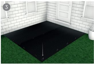
Lay your Cladco Weed Mat on top of the prepared soil, if you need to overlap ensure you do this with enough coverage for weeds not to penetrate through. Cover the weed mat with your desired coverage such as chippings, bark or stones so none of the weed mat material is exposed.
